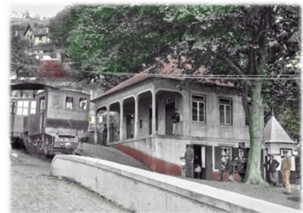
The Monte Station - built between 1911-1912 as part of the extension to Terreiro da Luta.
